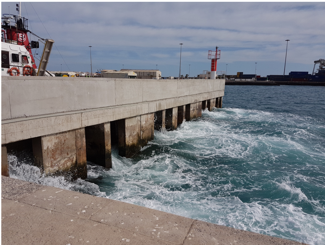
Image 3: Nowaves working under storm conditions in Las Palmas
