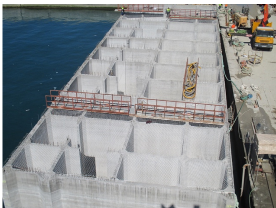
Image 1: Construction of NOWAVES technology caisson
